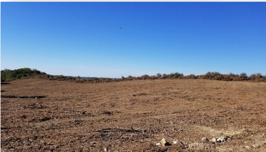
Figure 4. Cross-ripping at the 31.4-acre, Kentucky site. Note the intact forest in the background.
