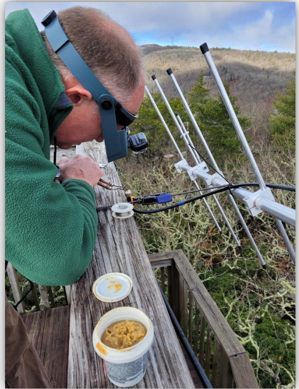
Figure 13. (Above) Kendrick Weeks, Western Wildlife Diversity Program Supervisor, solders a connector to a coaxial cable. Photo by Chris Kelly
