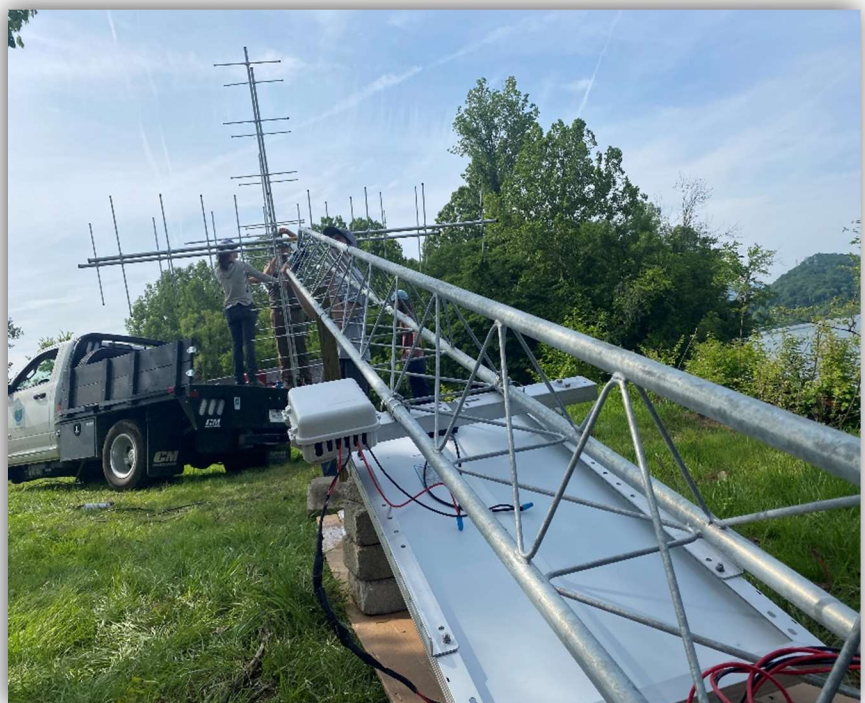
Figure 24. (Right) The Tennessee River Gorge Trust team installing a Motus tower. Photo by Eliot Berz/TRGT
